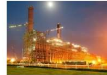
Steam Power Plants
