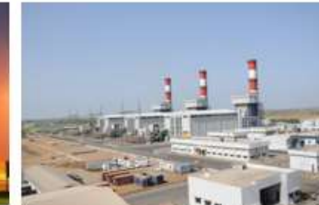
Gas Turbine Power Plants
