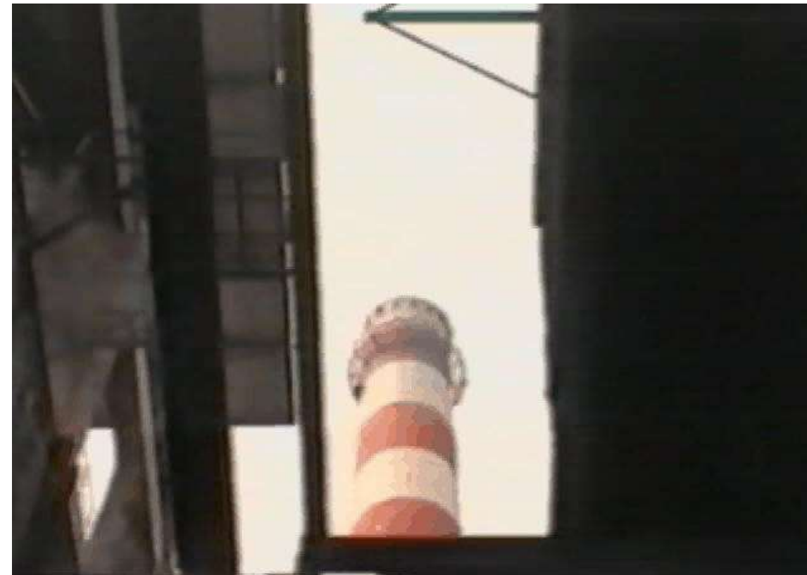
ESP energized during the startup of boiler with MOIS
