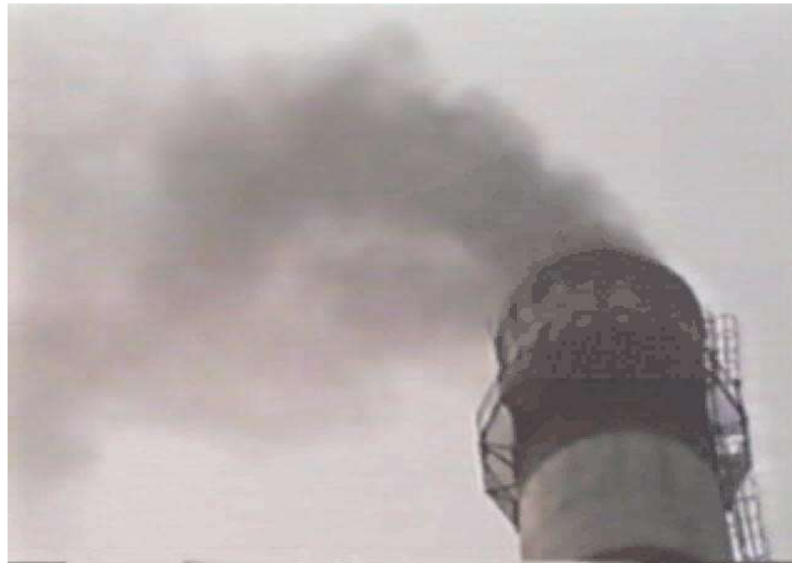
ESP de-energized during the startup of boiler with oil ignition
